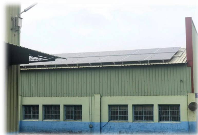
▲ The solar panels installed on the rooftop of our Taiwan factory
